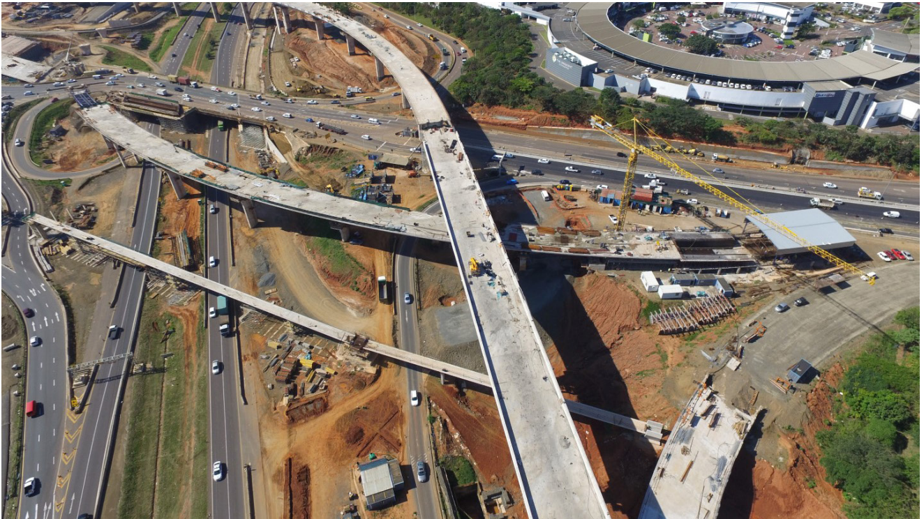
Fig. 4. uMhlanga interchange construction, Durban (Source: Caxton & CTP Printers and Publishers Ltd.)
