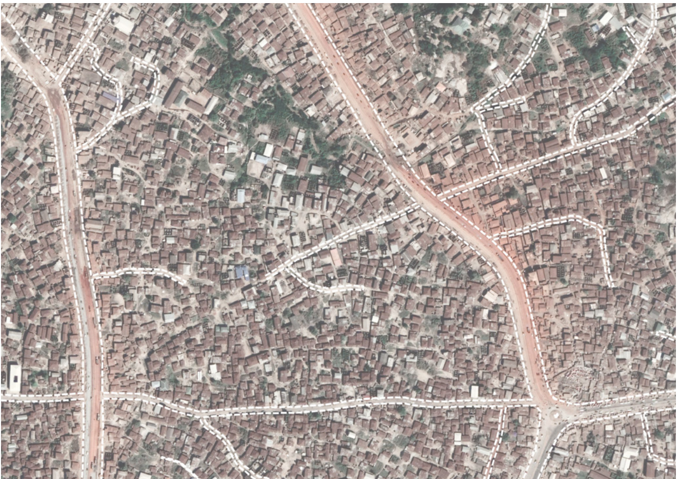
Fig. 11. Road widening in Old Abeokuta
