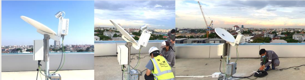
Vertical radar installation by Bangkok DSS intervention team
