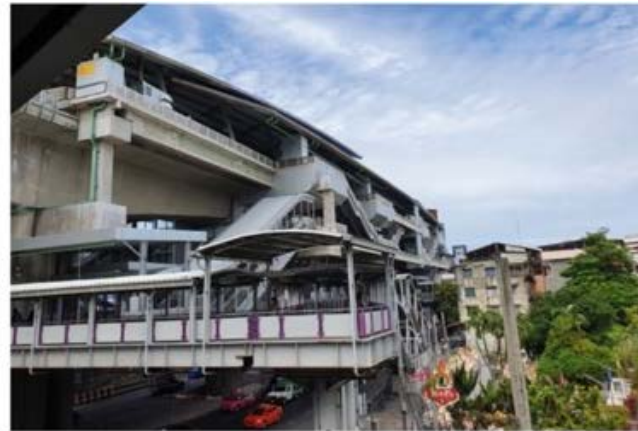
BTS Bang Wa Station
