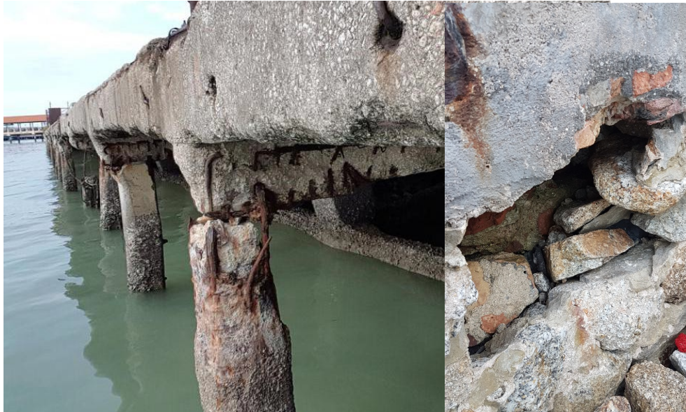
Dislodged blocks and structural issues at the Seawall
