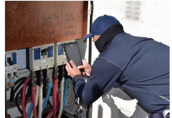
City of Cape Town official capturing performance data at a minisubstation for electricity asset management use case
