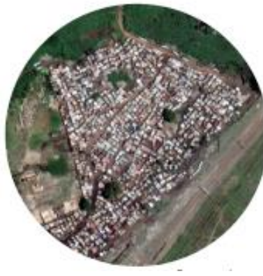
Figure 28: Emerging informal settlement within the floodline
